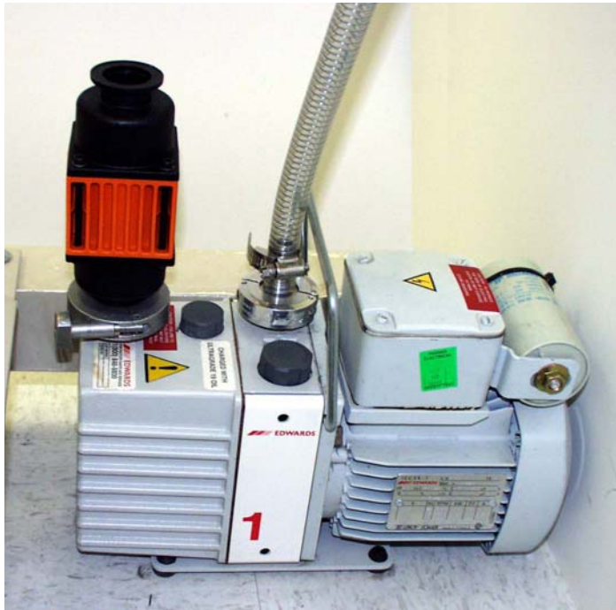
Figure 84 - Rotary Pump for the evacuation of the pump isolation valve
